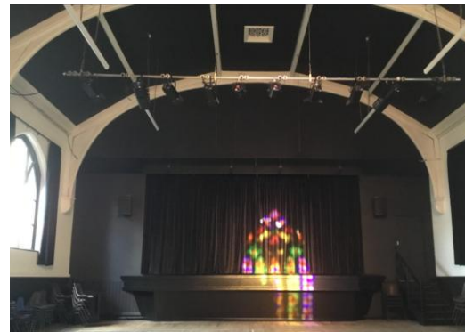
The Wesley Stage Works before and after
